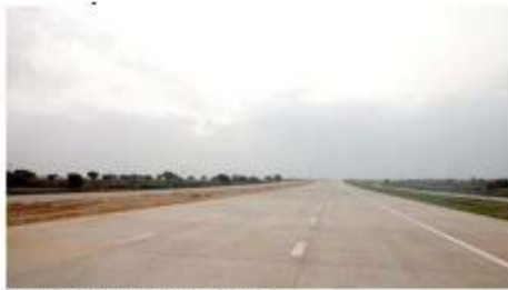
Fig.2. A view of rigid pavement.
