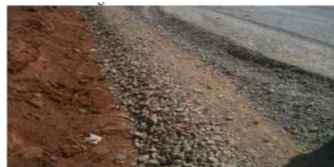
Fig.1. A view of Flexible pavement components.
