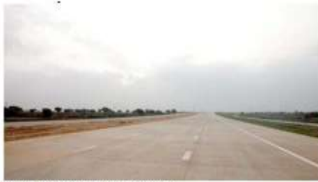
Fig.2. A view of rigid pavement.
