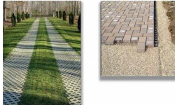
to infiltrate, treat, and enter the soil. Where they allow water to soak into a layer of rock, the amount of storm water and pollution reaching storm sewers and streams is greatly reduced. Permeable pavements Such as pervious concrete, permeable interlocking and porous asphalt. They are the best for commercial, residential and industrial areas but they are not recommended for streets, and highways.
