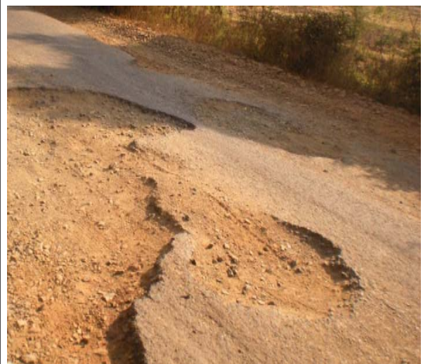
Figure 3: Photograph of the Existing Condition of the Study Road
